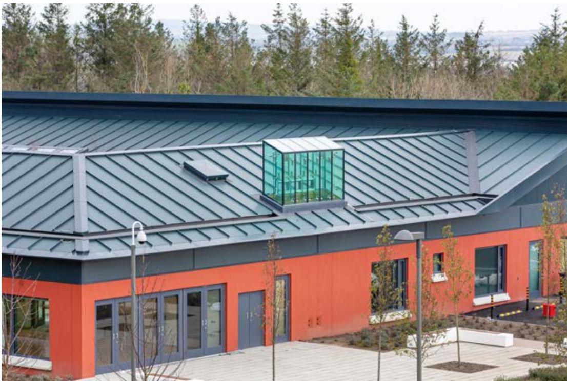
National Forensic Mental Health Servicen lasipilareilla varustettu lanterniini
